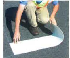
Fig. 2 Position PreMark® material according to diagram provided
