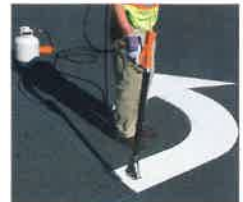
Fig. 3 Heat PreMark® material according to instructions.
