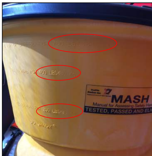
Figure 6b: Outside Sand Level Marks Shown
